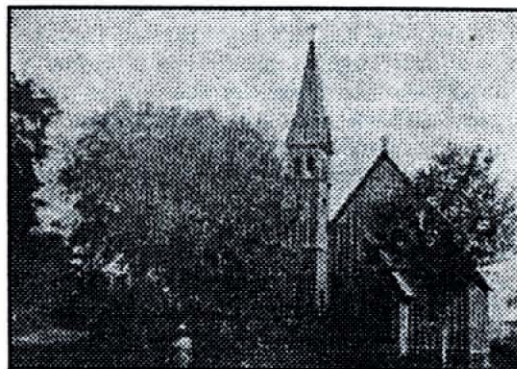
The Church of the Epiphany (Episcopal) in Allendale. Called the Chapel in the Willows from 1876-1894 when it stood near the NE corner of Franklin Turnpike and Cottage Place. The building was later moved to the NE corner of Franklin Turnpike and East Orchard Street.
